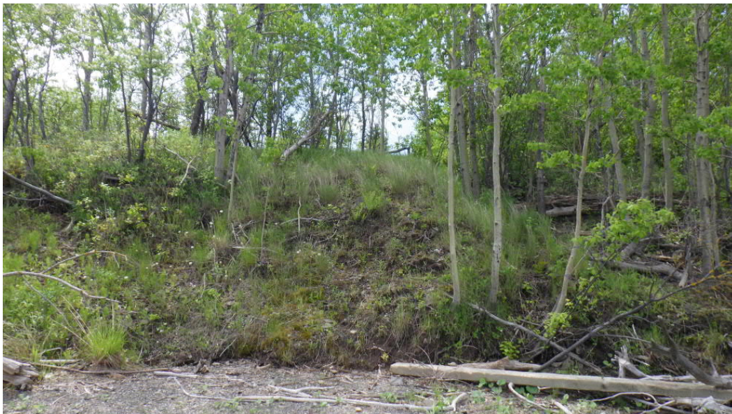
Photo 11: Eroding Coast North of NPNS Facility
